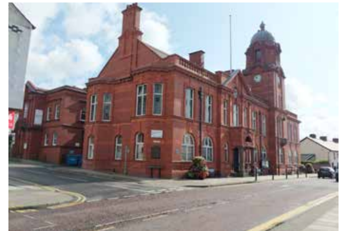
Westhoughton Town Hall is a heritage asset and a development opportunity
